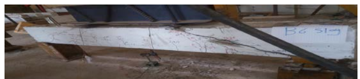
FIGURE30: CRACK DISTRIBUTION FOR S.S1 BEAM
