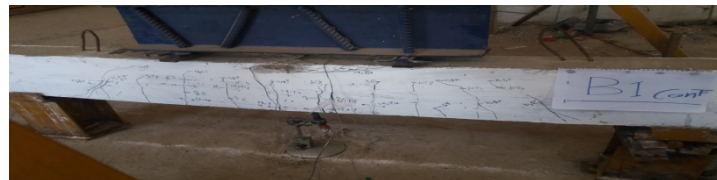
FIGURE26: CRACK DISTRIBUTION FOR NA BEAM
