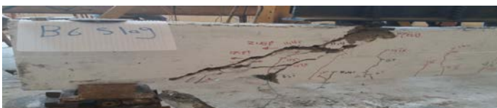
FIGURE36: SHEAR FAILURE FOR S.S1 BEAM
