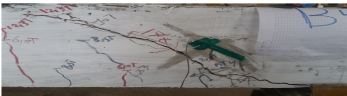
FIGURE35: SHEAR FAILURE FOR RAC1 BEAM
